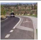
Raised cycle tracks are vertically separated from motor vehicle traffic. A raised cycle track may allow for one-way or two-way travel by bicyclists.
